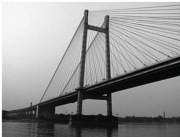
Fig. 18.11 Vidyasagar setu showing the long suspended deck standing on pylons
