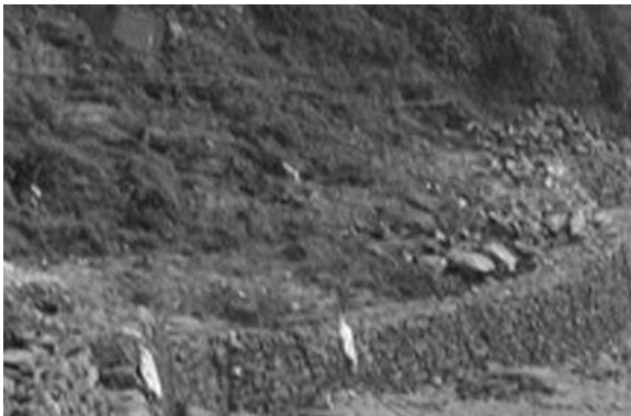
Fig. 21.28 Stabilization by stacked masonry wall
