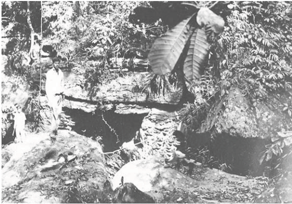
Fig. 22.2 Large sinkholes in limestone connected with subsurface solution channels
