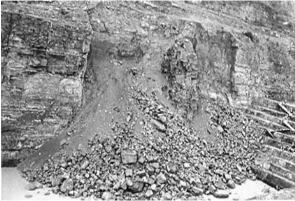
Fig. 21.19 Rock-cum-debris slide caused after slope cutting for construction purpose
