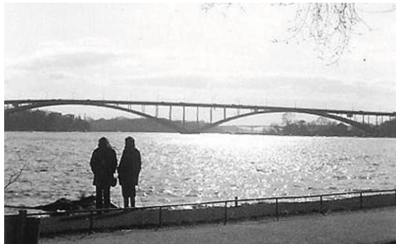
Fig. 18.7 Spandrel deck arch bridge with piers founded in river bed below water
