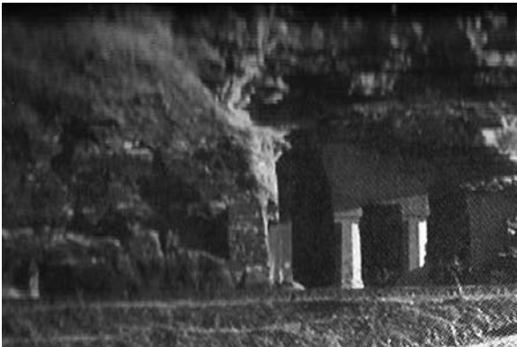
Fig. 4.1 Extensive deterioration of the cretaceous sandstones of Bagh Caves by chemical and mechanical weathering
