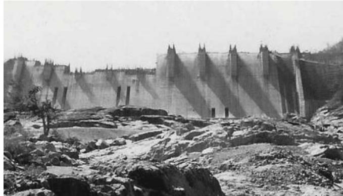
Fig. 14.24 Constructed concrete dam at the site on the river
