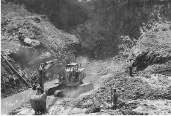
Fig. 14.10 Foundation preparation of rock-fill dam of the Salal project of Jammu and Kashmir
