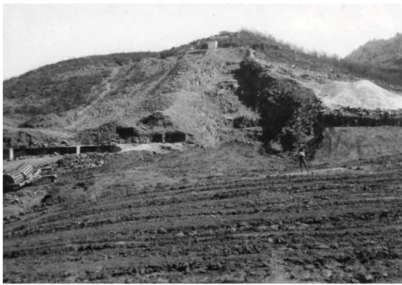
Fig. 14.28 Earth dam with layers of rolled earth
