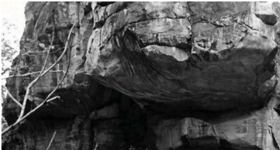
Fig. 3.20 Block joints in sandstone formed by sub-horizontal and vertical joints
