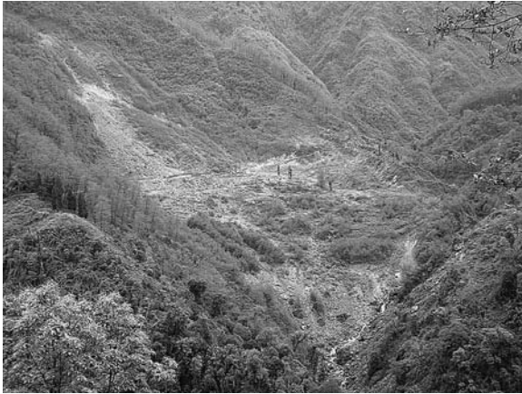
Fig. 21.17 Complex landslide (earthflow and debris slide) in Sikkim highway
