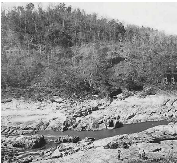
Fig. 14.23 A dam site on the North Koel river comprising fresh and massive granite gneiss before construction of a high concrete dam
