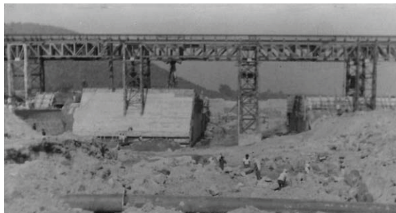
Fig. 18.14 A railway bridge on column and footing supports
