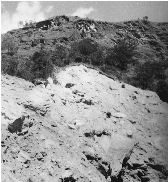
Fig. 21.12 Debris avalanche of loose overburden materials from a high hill
