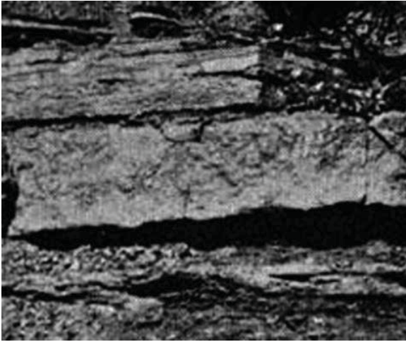
Fig. 2.11 Limestone beds showing solution effect along the bedding plane (see also Fig. 22.2)
