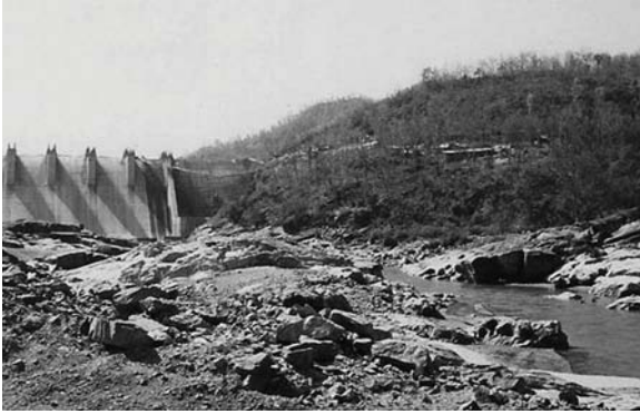
Fig. 14.14 Spillway with chute and discharge of water to the downstream part of North Koel concrete dam (see full view of dam in Fig. 14.24)
