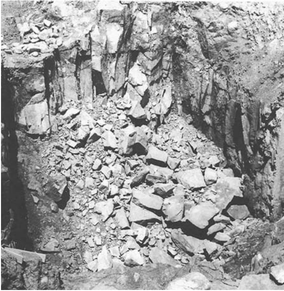
Fig. 21.4 Rock fall of jointed rocks, the failure surfaces being mostly vertical
