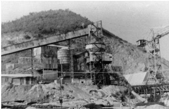
Fig. 14.27 A batching plant where aggregates and cement are mixed in fixed proportions to make concrete of design strength
