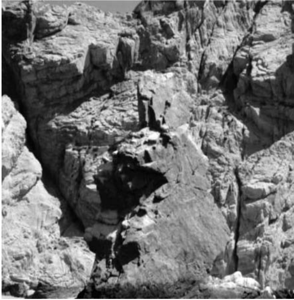
Fig. 4.8 Widening of rock joints and cracks, which may crumble the entire rock mass (a slip plane is seen along a joint plane in the front)
