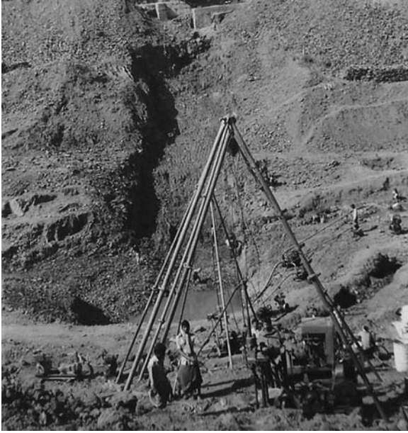
Fig. 11.18 Rock drilling by drill rig
