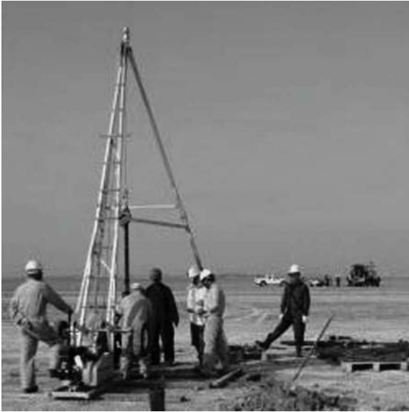
Fig. 11.14 Subsoil exploration by borehole with sampler tube
