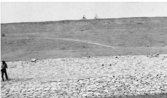
Fig. 14.12 An earth dam immediately after compaction of earth and stone pitching
