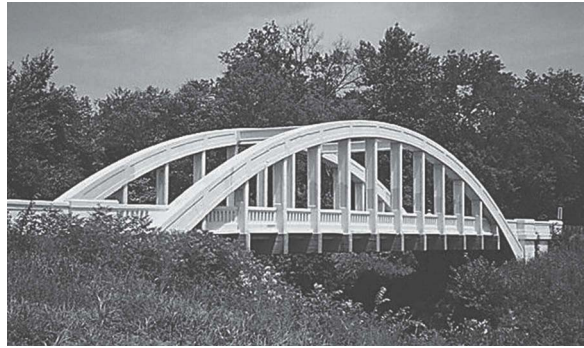
Fig. 18.5 An arch bridge
