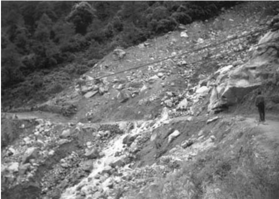
Fig. 21.29 Disruption of highway in Darjeeling by a huge landslide of hill slope after heavy rains and snow
