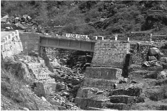
Fig. 18.1 A single-span steel beam bridge constructed over a high-altitude stream
