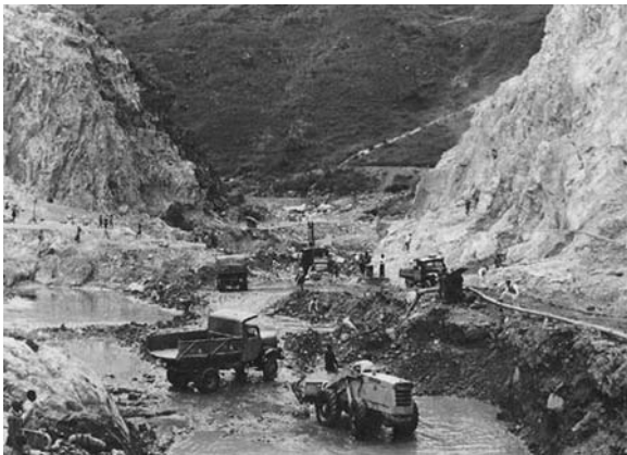
Fig. 14.26 Removal of river detritus after diversion of river
