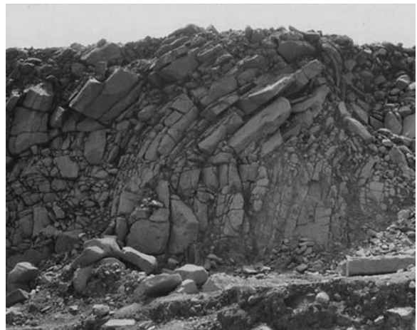
Fig. 21.6 Topple of rock blocks from a dam abutment along multiple joint planes
