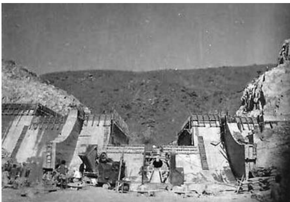
Fig. 14.3 Concrete gravity dam under construction across the river Umiã, Meghalaya
