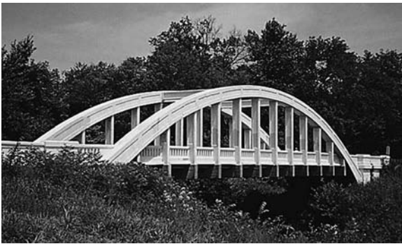
Fig. 18.5 An arch bridge
