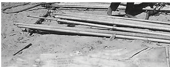
Fig. 13.8 Drill rods for injecting grout
