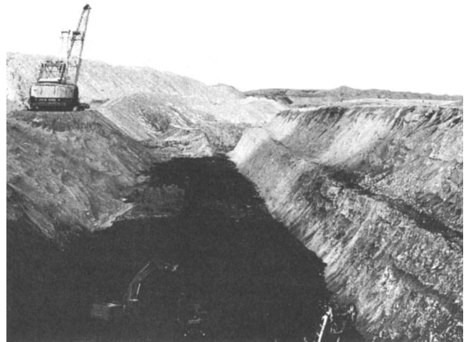
Fig. 14.3.1.6. Dragline on the spoil side.
