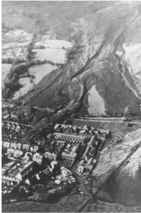
Figure 7.4 Mudflow from a spoil heap at Aberfan, South Wales, October 1966.
