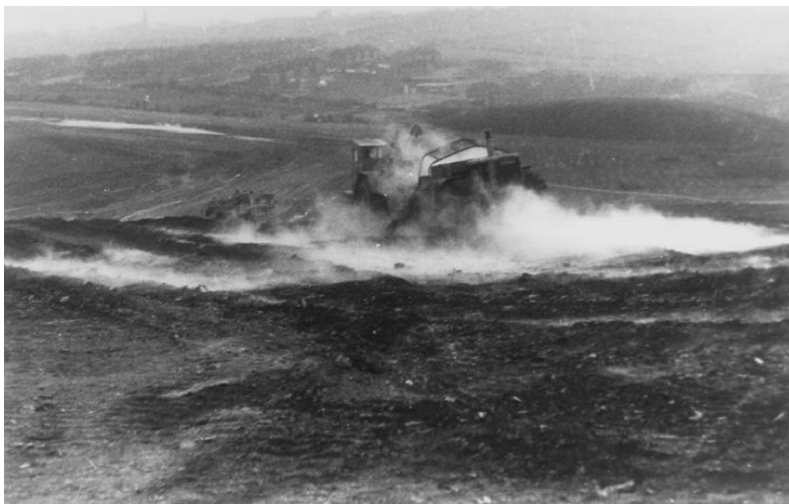
Figure 7.3 Levelling spoil over a hot spot caused by spontaneous combustion, Barnsley, England.
