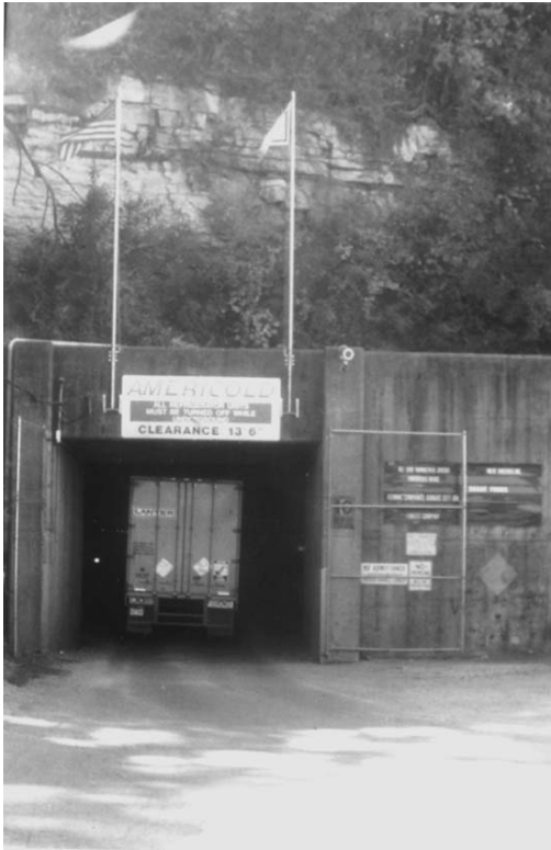
Figure 1.1 An entrance to old workings in the Bethaney Falls Limestone, Kansas City, United States, which are now used for warehousing, cold storage etc.
