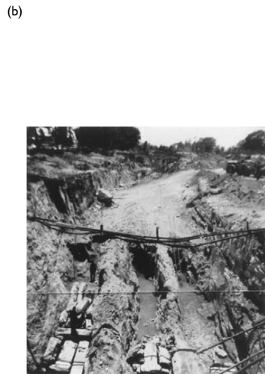
Figure 4.15 (a) Plugging reef outcrops with concrete. (b) Stabilization of shallow outcrop of three adjacent stopes by a concrete plug.
