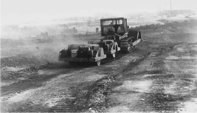
Figure 7.14 Compacting spoil with a vibratory roller.
