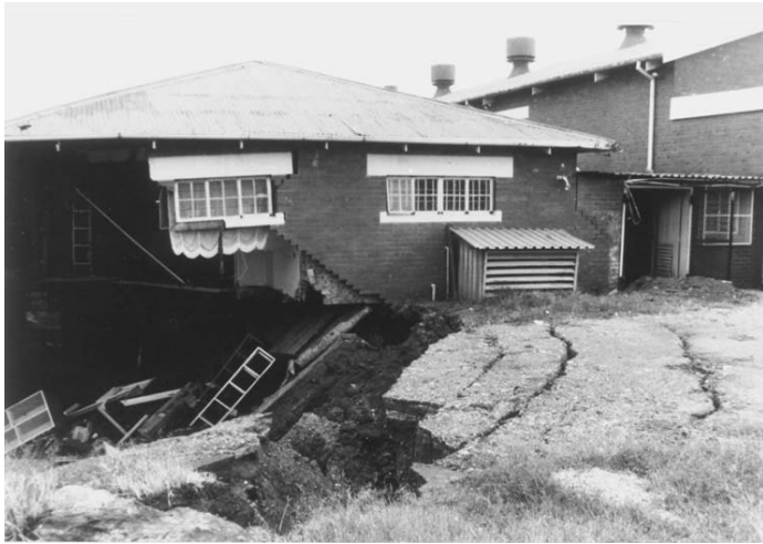
Figure 5.7 A sinkhole formed in deposits overlying the Transvaal Dolomite, south of Pretoria, South Africa.
