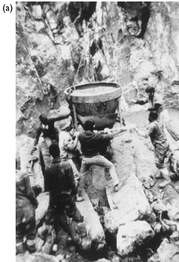
Figure 4.15 (a) Plugging reef outcrops with concrete. (b) Stabilization of shallow outcrop of three adjacent stopes by a concrete plug.
