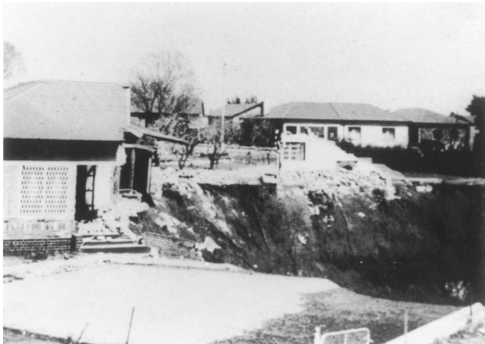
Figure 5.8 A sinkhole developed at Blyvooruitzicht that claimed five lives.
