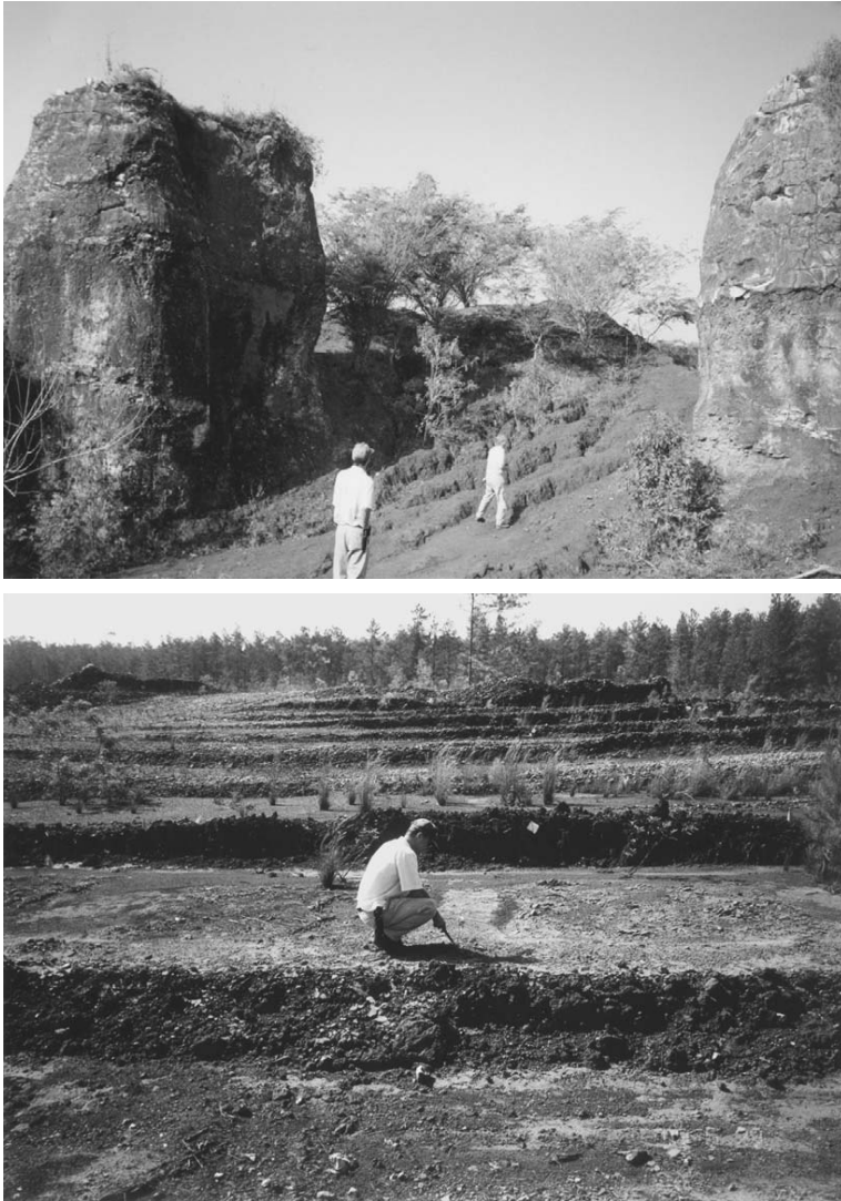
Figure 6.23a Rehabilitation of the Las Mercedes open-pit bauxite mine providing land for forestry, Pedernales, Dominican Republic, West Indies; showing abandoned mine workings and remnant limestone pillars (upper), reforestation and restoration (lower).
