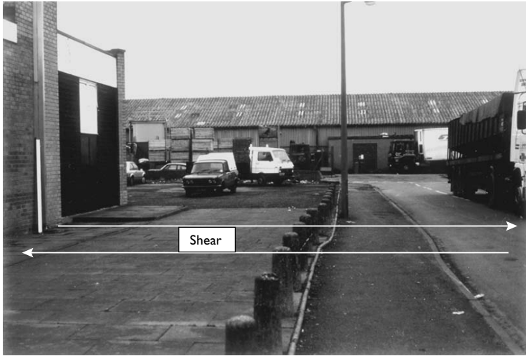
Figure 3.37 The reactivation of the Hollybush Fault, Newstead, Staffordshire, showing later 0.1–0.3 m lateral shear of the kerbstones, pavements and buildings, with no observable vertical displacement.
