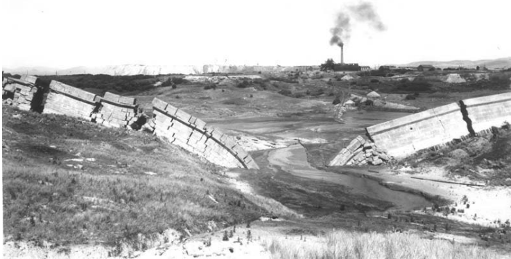
Figure 4.6 Subsidence, up to 20 m in places, above Hodbarrow Mine, Millom, Cumbria. (Reproduced by kind permission of the British Geological Survey. © NERC. All rights reserved. IPR/61–05C.)
