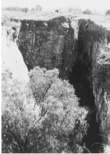
Figure 4.13 Collapse of surface outcrop of a reef into stope.
