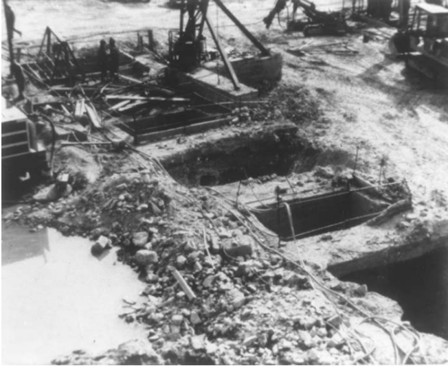
Figure 4.23 Sinking of winces on stopes at Standard Bank site.
