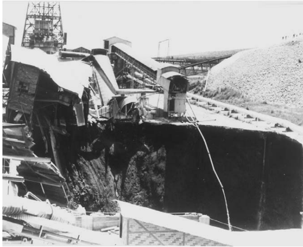
Figure 5.27 A sinkhole which engulfed a three-storey crusher plant at West Driefontein Mine, Far West Rand, and claimed 29 lives.
