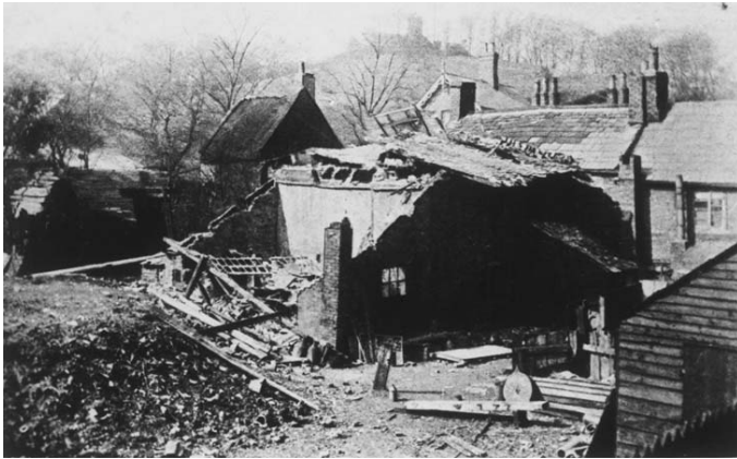
Figure 5.20 Catastrophic damage caused by bastard pumping of salt brine, Cheshire, England. (From Calvert, A.F. 1915. Salt in Cheshire , Spon, London.)
