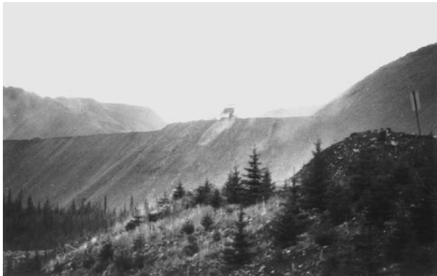
Figure 6.22b Restoration by end-tipping of waste into old open-pit coal workings, near Lethbridge, British Columbia.
