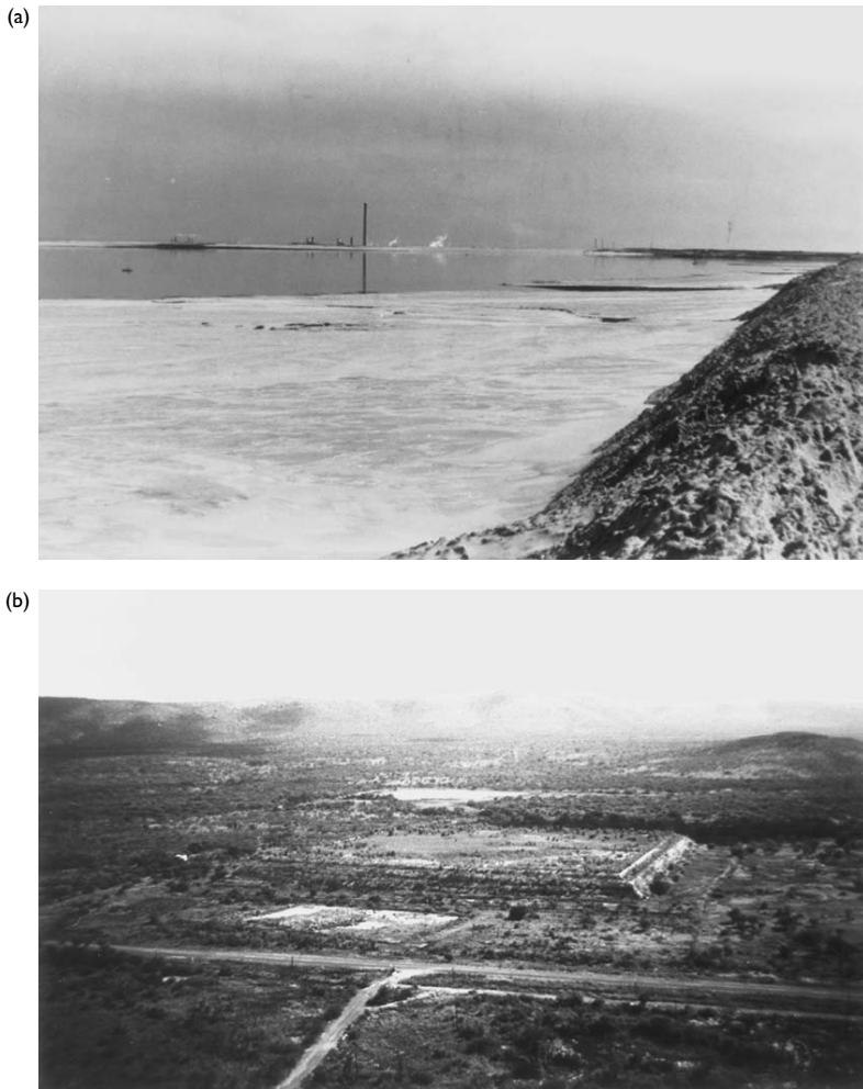
Figure 7.5 (a) Part of a large tailings facility at Athabasca Tar Sands, Fort McMurray, Alberta, showing dam, beach and lagoon. (b) A ring tailings dam at a tin mine in North West Province, South Africa.
