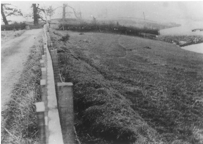
Figure 5.19 Subsidence caused by wild brine pumping, Cheshire, England. Note the tension scar to the right of the fence and the flash in the top right-hand corner.
