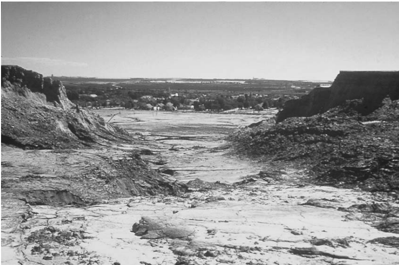
Figure 7.11 Failure of the Merriespruit tailings dam, South Africa, showing lobate flowslide. (Courtesy of Professor Dick Stacey & SRK Consulting South Africa.)
