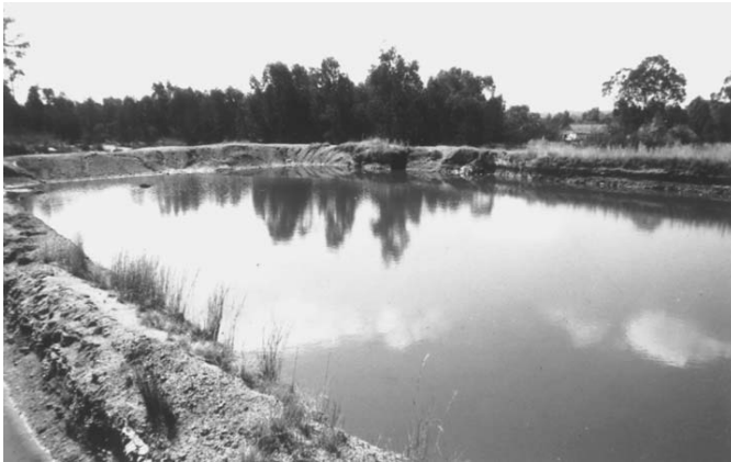
Figure 8.15 Pollution control pond, one of four.
