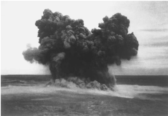
Figure 10.3 Extinguishing mine fire by directional blasting in the south fire area of Beishan Coalfield, Qitai County, China.
