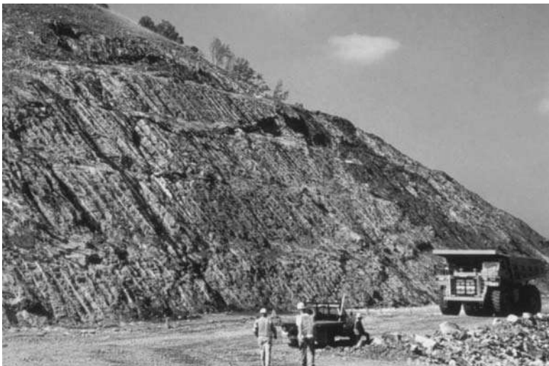
Figure 11.10 Example of controlled blasting for rock cut on highway project (strong, highly folded gneiss, I-26/US23, near Mars Hill, North Carolina) (courtesy: North Carolina Department of Transportation).
