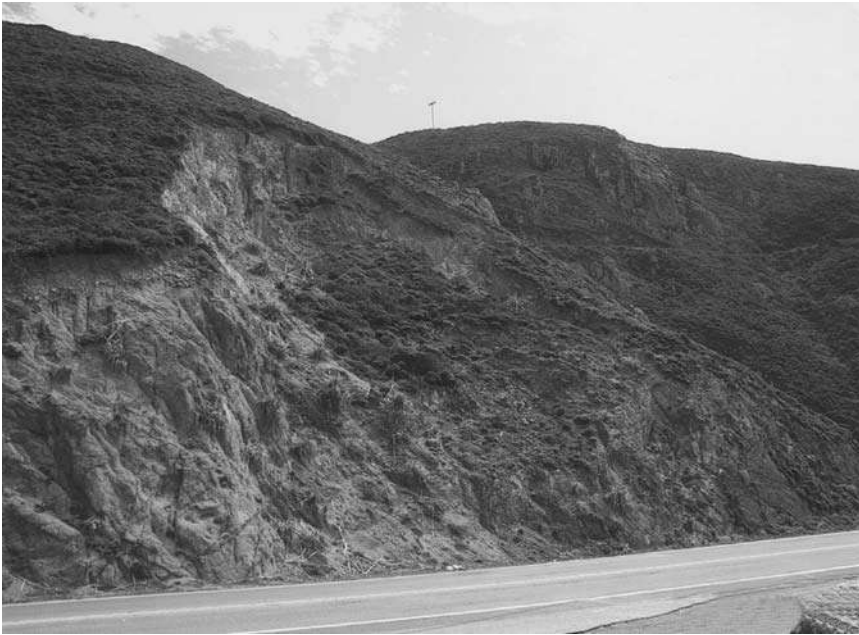
Figure 8.1 Circular failure in highly weathered, granitic rock (on Highway 1, near Devil's Slide, Pacifica, California).
