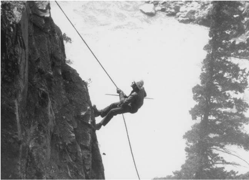
Figure 12.18 High scaler suspended on rope and belt while removing loose rock on steep rock slope (Thompson River Canyon, British Columbia, Canada) (TRB, 1996).
