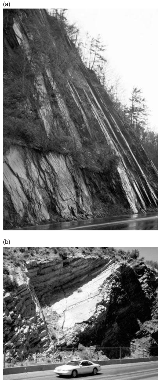
Figure 2.1 Rock faces formed by persistent discontinuities: (a) plane failure formed by bedding planes parallel to face with continuous lengths over the full height of the slope (shale on Route 19 near Robbinsville, North Carolina); (b) wedge failure formed by two intersecting planes dipping out of the face (sedimentary formation on Route 60 near Phoenix, Arizona).
