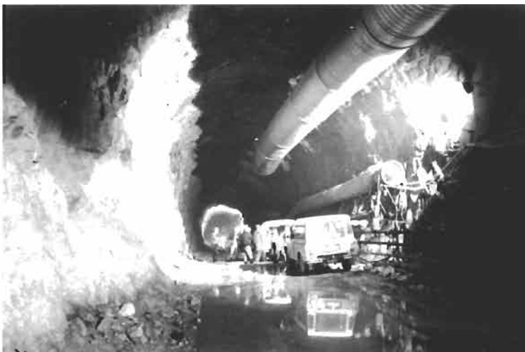
Figure 1.11 Hydroelectric cavern in Portugal.
