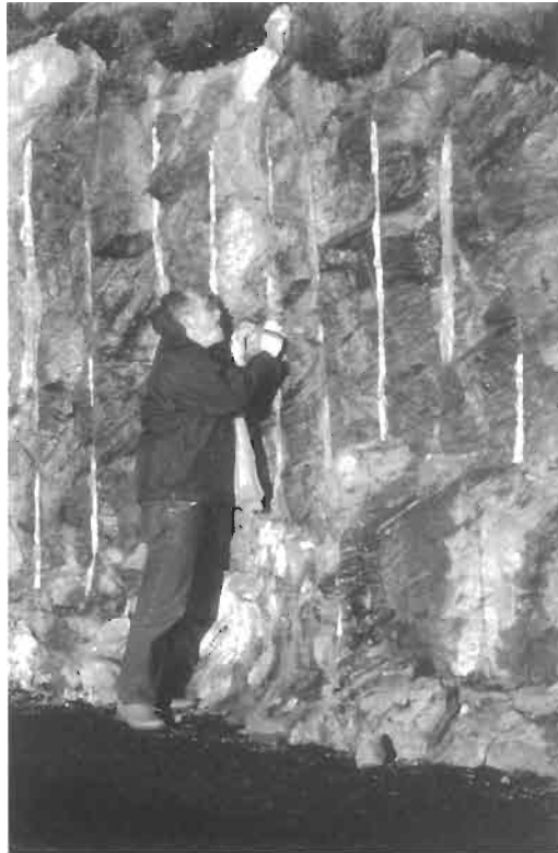
Figure 15.16 A static pre-split formed using expanding grout (Isle of Lewis, Scotland).
