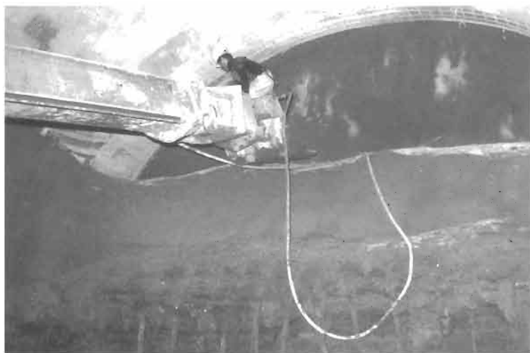
Figure 16.9 Construction of the Bochum metro in Germany.
