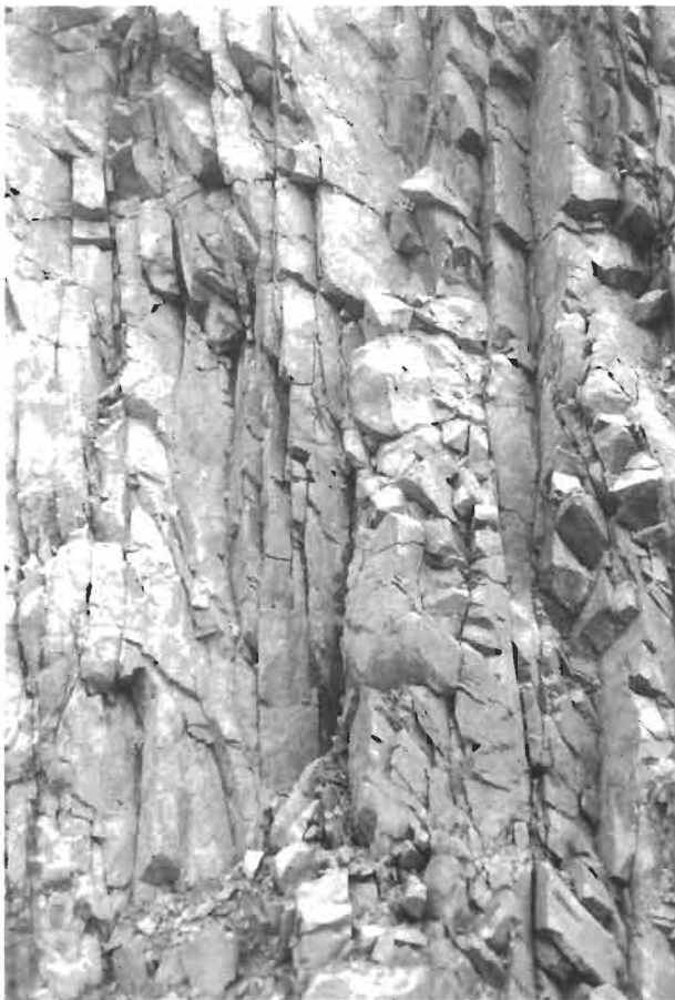
Figure 2.3 Zone of highly fractured rock.
