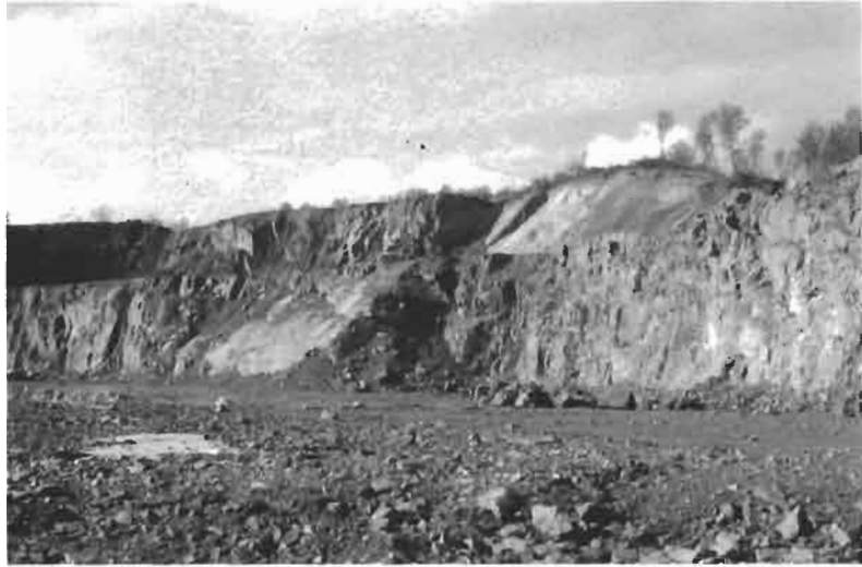
Figure 1.8 Open-pit mine with slope instabilities.
