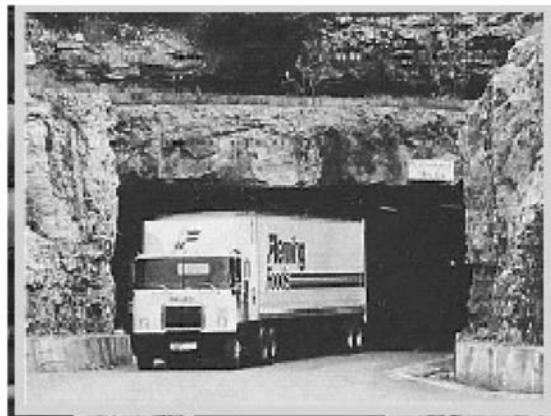
Figure 15.6 Some underground facilities – a network of excavations of various kinds.
