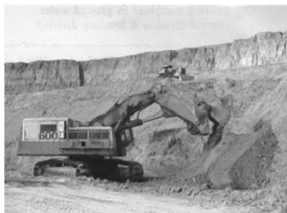
Figure 6.7 A hydraulic excavator working at Civil site.
