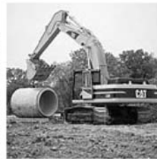
A hydraulic excavator
