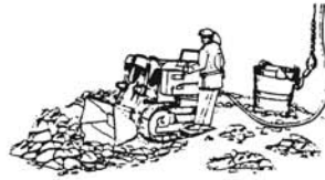
(b) Eimco-630 loader mucking from sinking shafts & development faces
