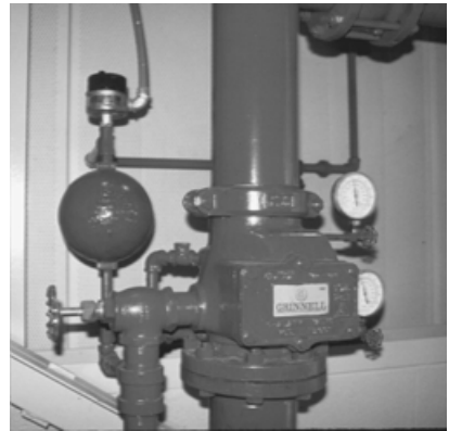
FIGURE 6.35 Wet-pipe sprinkler valve.
