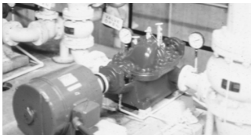
FIGURE 6.71 Fire pump, electric, horizontal shaft.
