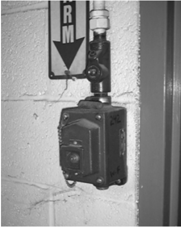
FIGURE 6.11 Pull station for hazardous location.
