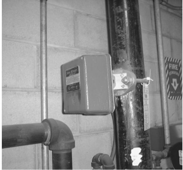
FIGURE 6.39 Flow switch.
