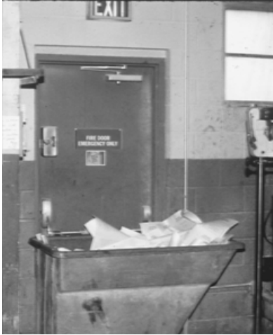
FIGURE 4.4 Obstructed exit.
