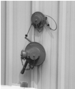
FIGURE 6.77 Wall hydrant.
