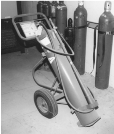
FIGURE 7.17 Wheeled carbon dioxide extinguisher.
