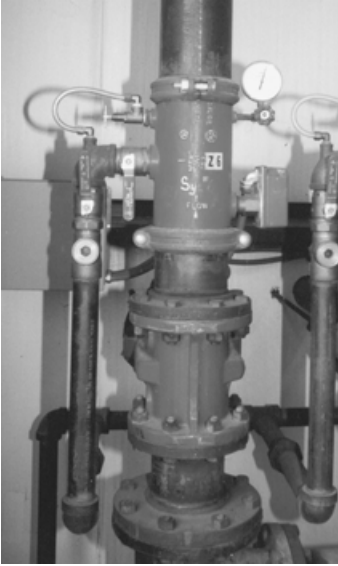
FIGURE 6.34 Wet-pipe sprinkler without valve.
