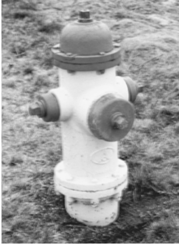
FIGURE 6.75 Dry barrel hydrant.
