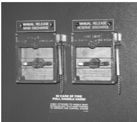
FIGURE 6.87 Carbon dioxide system manual trip.
