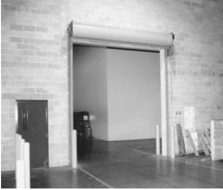
FIGURE 6.2 Fire door, overhead rolling.
