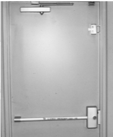
FIGURE 4.7 Locked exit.
