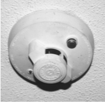
FIGURE 6.15 Combination smoke and heat detector.
