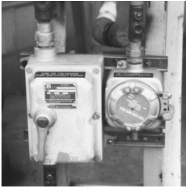
FIGURE 5.30 Explosion-proof control box.
