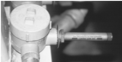
FIGURE 6.81 Carbon dioxide system heat detector.
