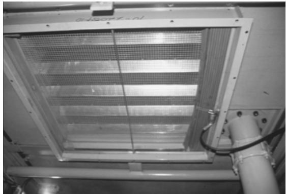
FIGURE 6.86 Carbon dioxide system vent closer.
