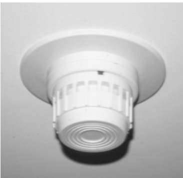
FIGURE 6.14 Heat detector.
