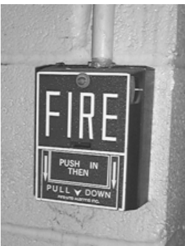
FIGURE 6.10 Pull station with tamper-resistant cover.
