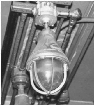
FIGURE 5.27 Explosion-proof light, incandescent.
