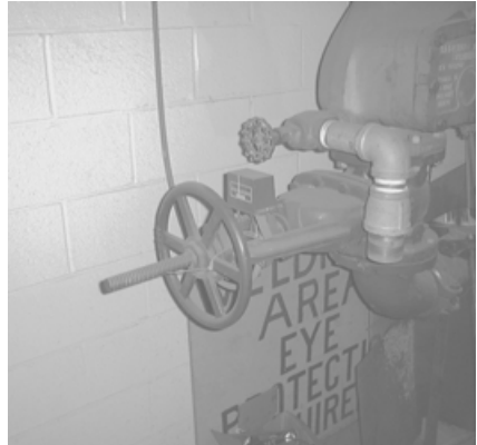
FIGURE 6.54 Outside screw and yoke (OS & Y) valve.
