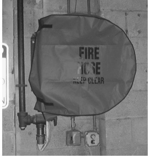
FIGURE 6.25 Standpipe hose station, class II.
