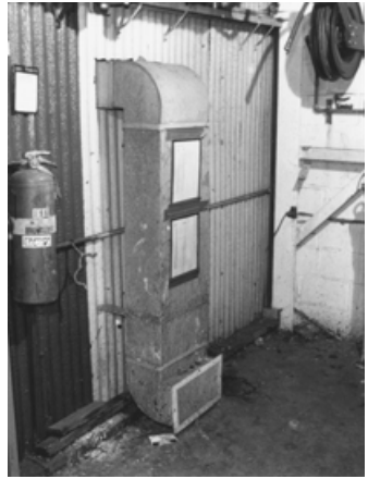
FIGURE 5.26 Floor level ventilation.
