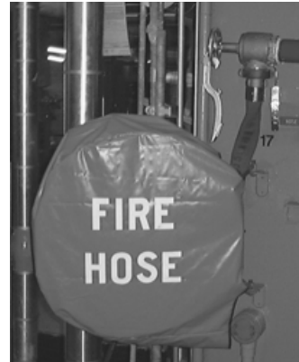
FIGURE 6.24 Standpipe hose station, class I.
