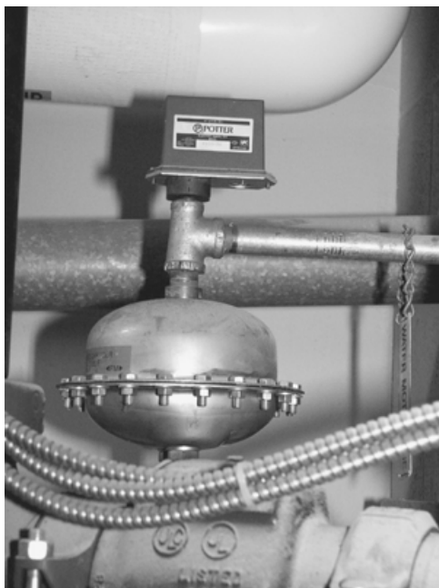
FIGURE 6.38 Pressure switch.
