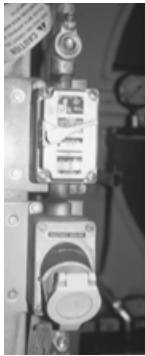
FIGURE 5.31 Explosion-proof outlet.
