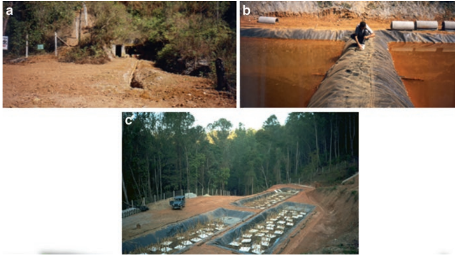
Fig. 6.8 The ARUM system in Brazil. (a) The portal of the abandoned gold mine. (b) The precipitation ponds. (c) Cattails transplanted to Styrofoam™ floats as living cover for ARUM cells. Photograph shows initial system. Which was later replaced (Kalin & Caetano Chaves, 2003). (Photographs by Boojum Research)
