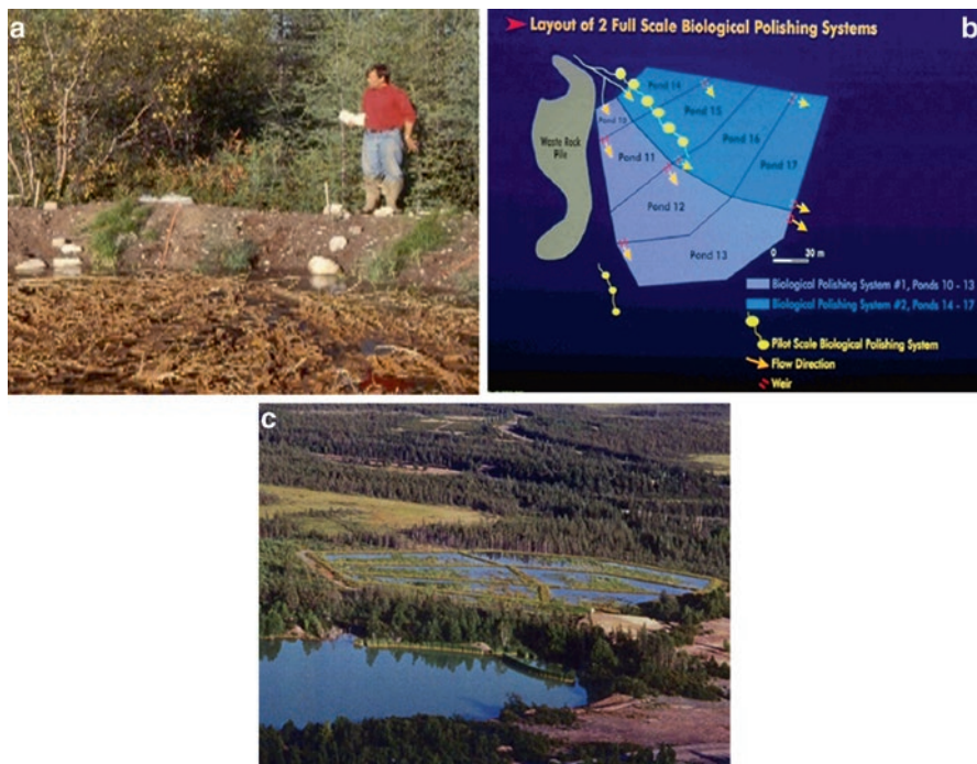
Fig. 9.4 (a) Martin Smith, a Boojum researcher, working on one of the pilot ponds. Note brush in the pond, used as a substrate for periphyton growth. (b) A schematic showing the pilot-scale ponds in yellow, and the scale-up in blue. The series of 6 yellow circles extending through pools 14 and 15 were the pilot ponds which served as design criteria for the scale up. First to be scaled up were pools 10–13 (in lighter blue), followed later by pools 14–17 (darker blue). Yellow arrows denote direction of flow. The three yellow circles in the lower left were ARUM test cells treating the drainage from the waste rock pile. Organics were added to a completely rust-covered sphagnum bog. (c) Aerial photograph of the OEP and polishing ponds in the meadow below the OEP. All photographs by Boojum Research.
